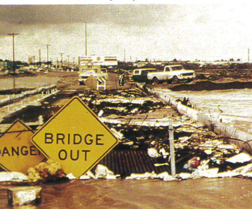
Only two Salt River bridges withstood 1980's 55-year flood.
